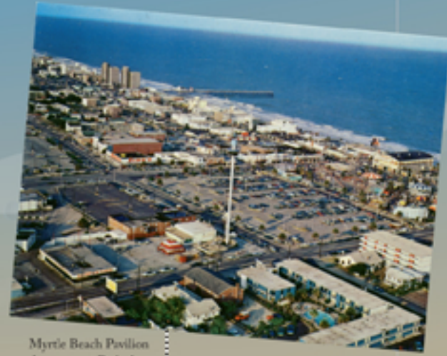
Myrtle Beach Pavilion Amusement Park closes and is demolished
